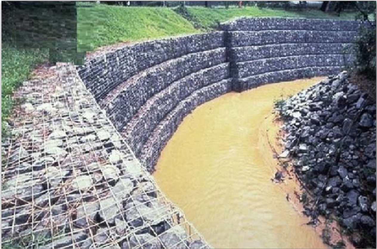
Fig 10.7 Gabion basket placed at river bend to prevent river bank erosion during flooding
