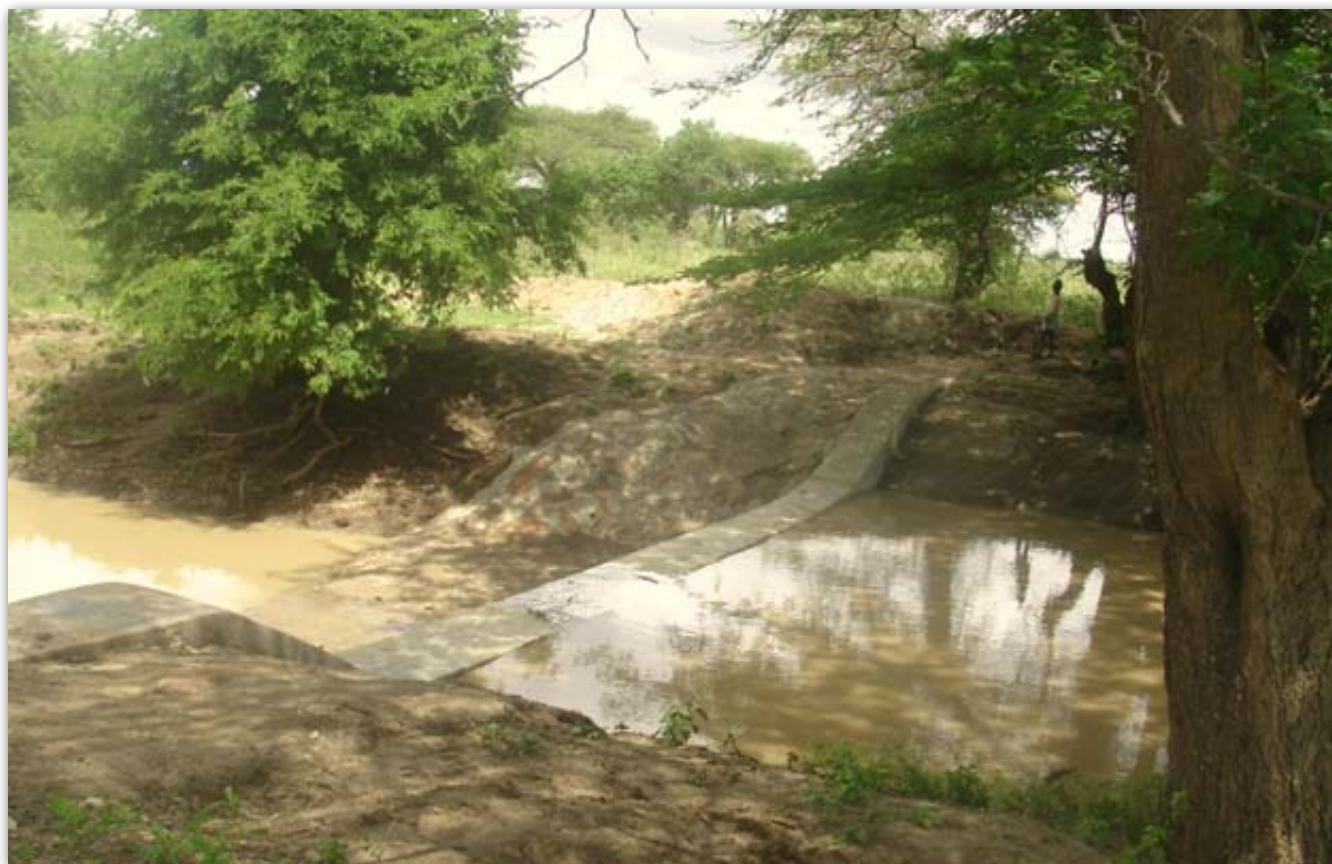
Fig 13.2 Typical masonry sediment storage dam (Kotido)
