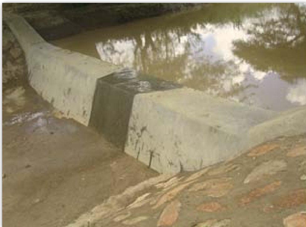
Fig 14.3 Good overflow spillway masonry dam
