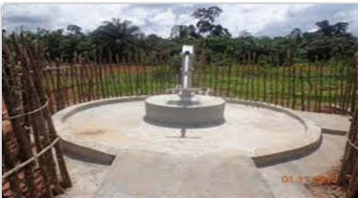
Fig 15.6: Shallow well with proper area drainage system
