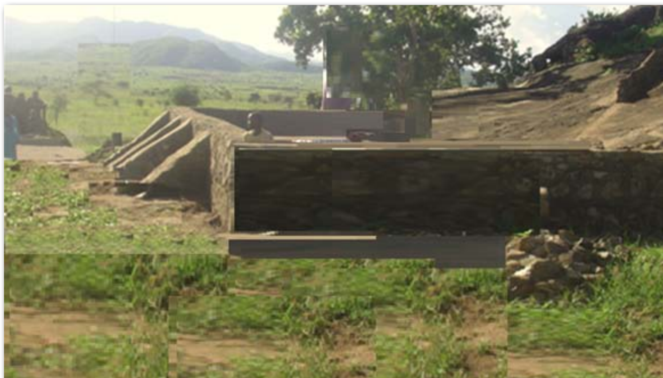
Fig 5.1 Rock catchment runoff water harvesting (Kotido)
