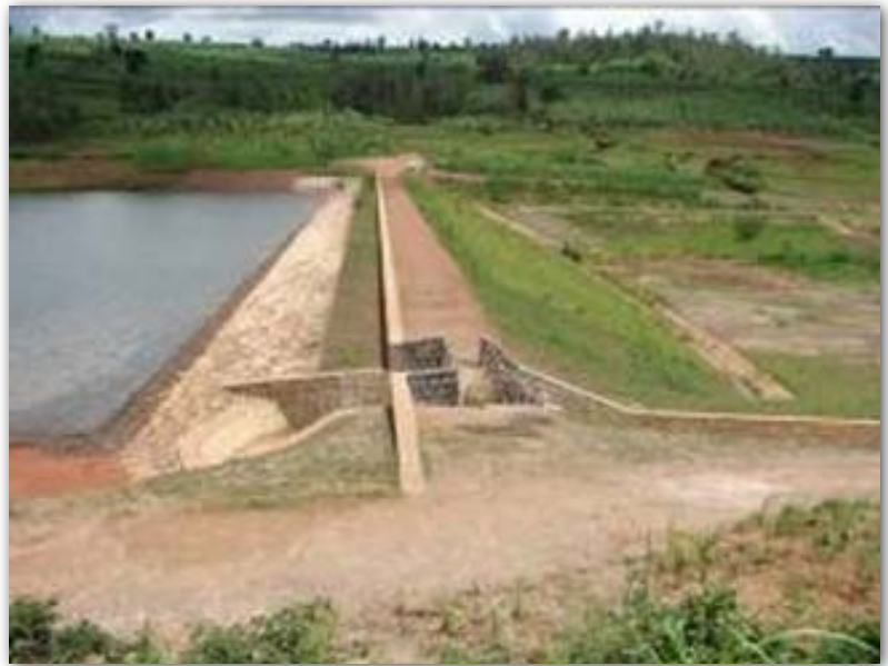
Fig 12.1 Typical view of zoned earth embankment dam
