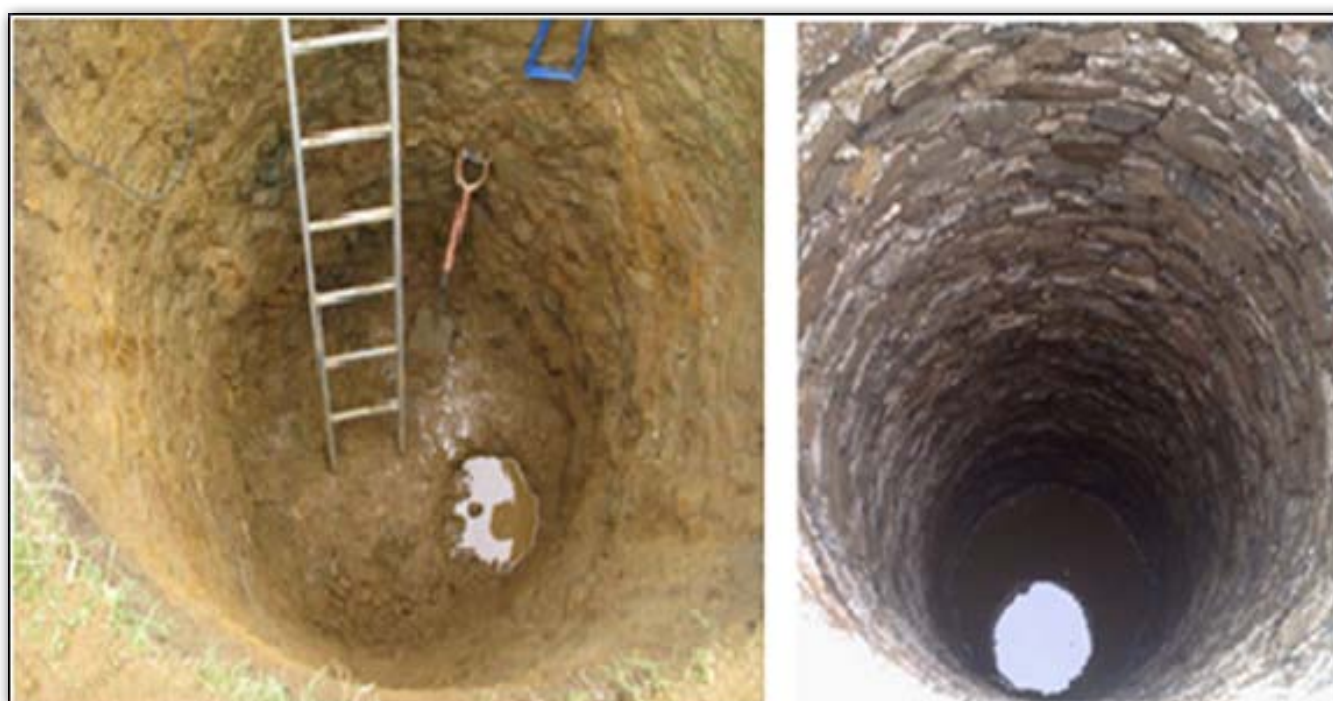
Fig 15.5: Manual hand dug well construction
