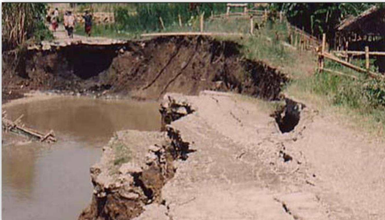
Fig 10.3: River bank collapse, caused by erosion, affects livelihoods of community
