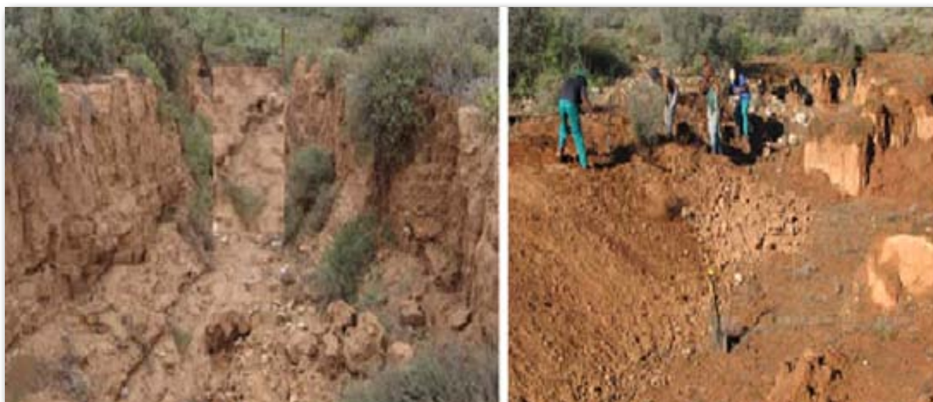
Fig 2.6 Reshaping vertical and deep gully
